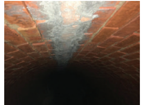
Grouted repair of cracked crown.
