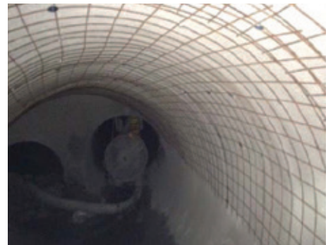
Welded wire mesh placed across crown of pipe after initial GeoSpray application.
