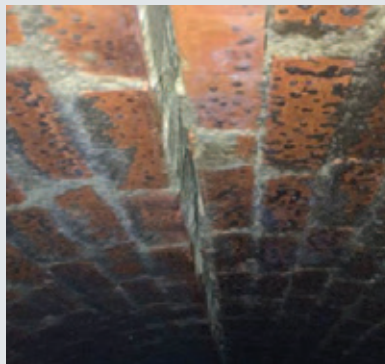
Close up of damaged brick crown.
