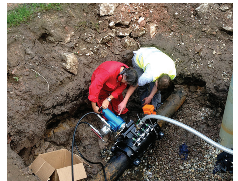
Cutting tool is leveled and prepped for milling.
