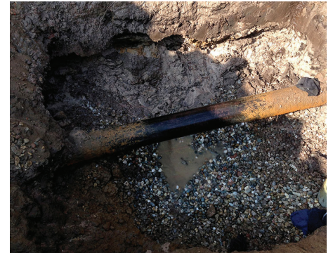
Excess Water is drained, pipe is thoroughly cleaned and prepped for valve body.
