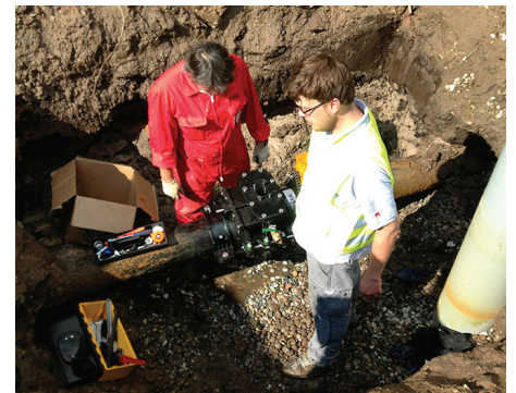
Wedge gate is lowered and drip tight seal is created.
