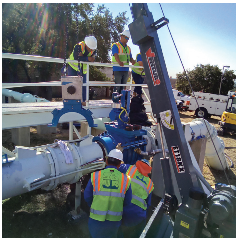
The gearbox was secured to the pipe.
