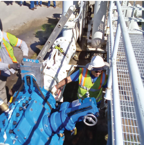
The EM machine then milled a 120° slot across the top of the pipe.
