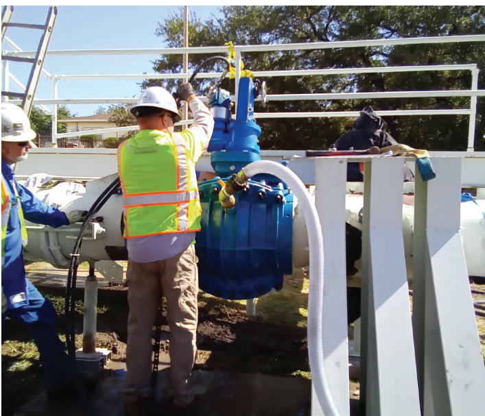
The blow off hose carried swarf created from the milling, away from the water inside the pipe.
