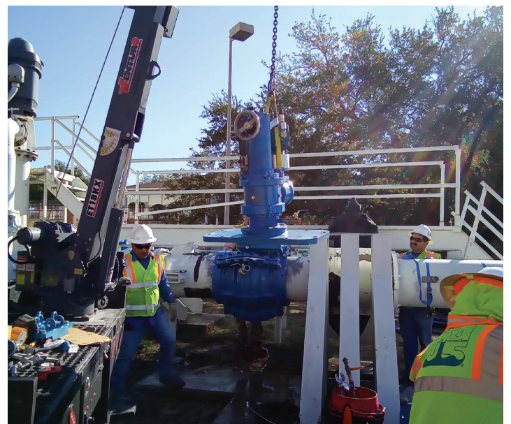
With the integral gate closed, the EM machine was removed.
