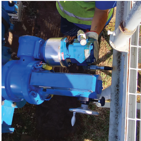
The EM machine then milled a 120° slot across the top of the pipe.
