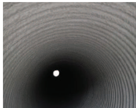
Completed GeoSpray geopolymer lining.
