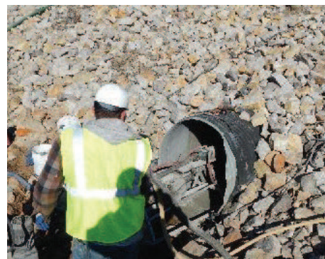
Completing first GeoSpray lining pass.
