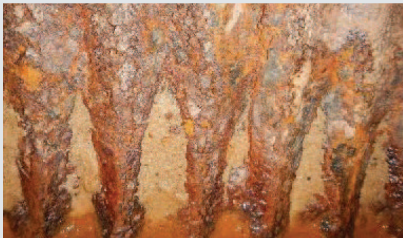
Corroded culvert prior to rehab.
