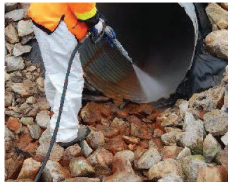
Pressure washing loose material from culvert.
