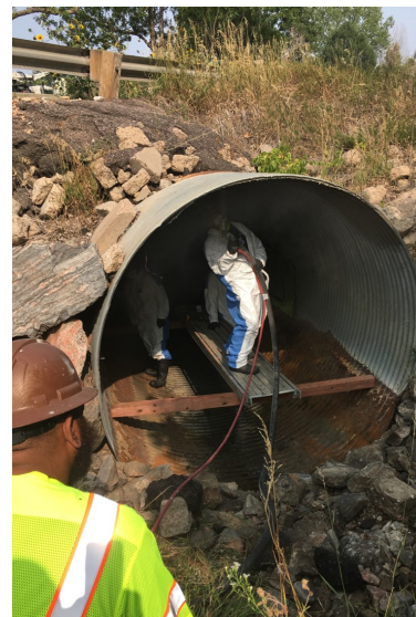
Due to the size of the culvert, GeoTree's GeoSpray geopolymer was hand spray applied.
