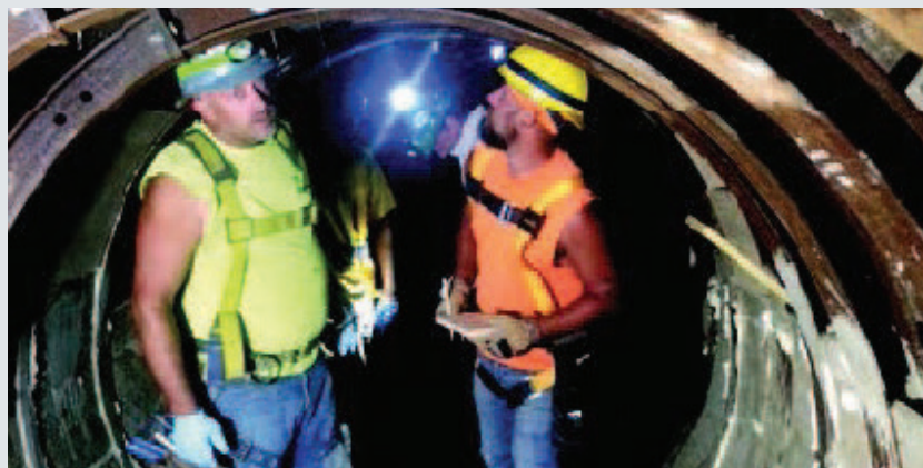
Installation of lagging around and behind ribs.
