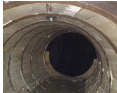
Completed installation of the ribs and lagging.
