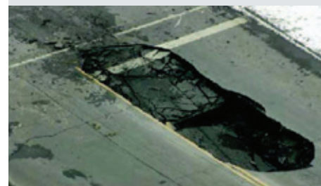
Sinkhole on Tireman Avenue caused by damaged interceptor.
