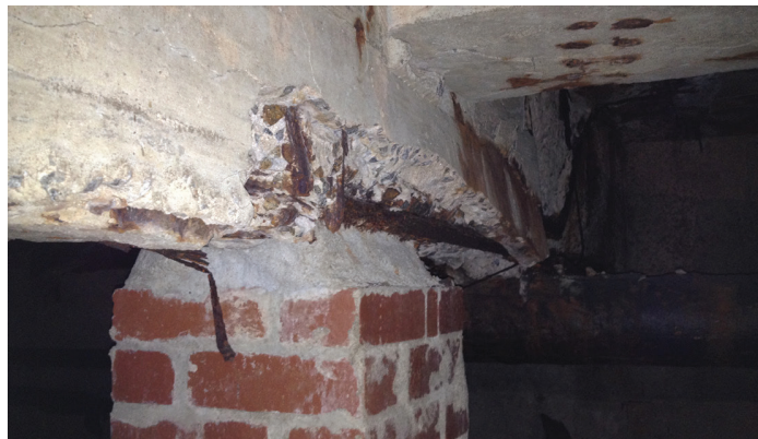
Deteriorated beam prior to repair
