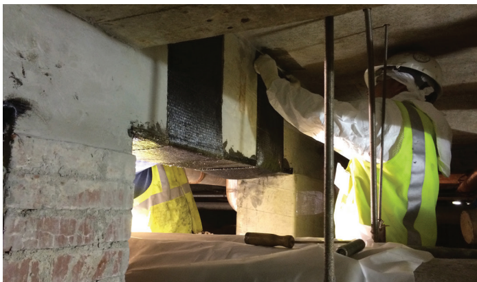
Installing U-wraps
