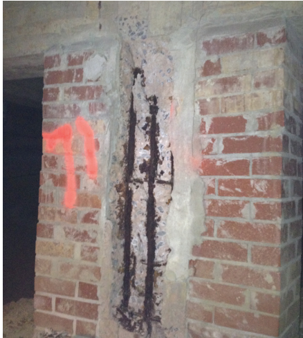
Deteriorated column prior to repair
