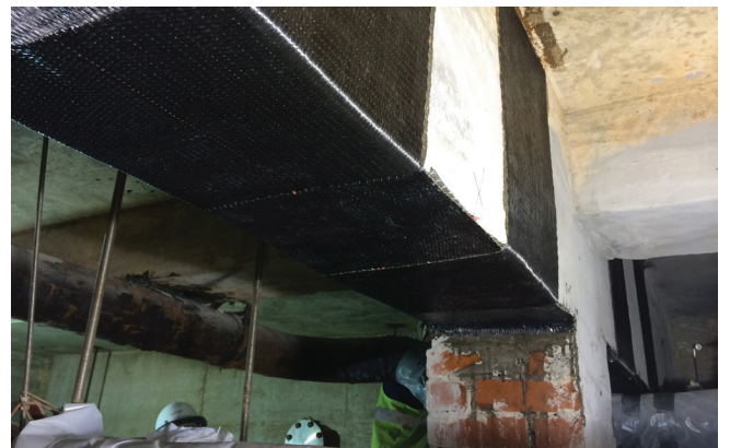
Flexure plies and U-wraps
