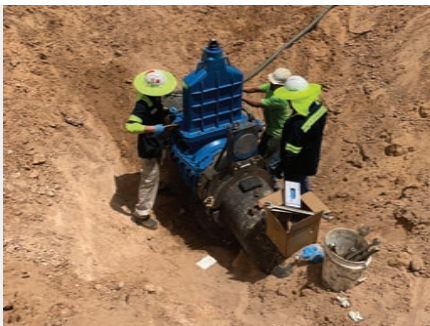
6 Installing the bonnet
