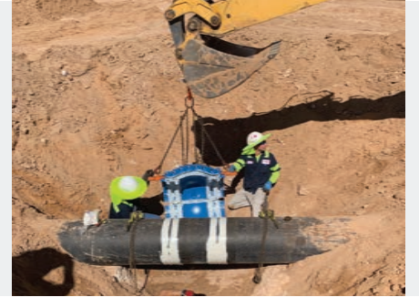
2 Fitting the bottom (part B) of the AVT EZ Valve
