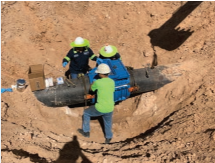
3 Fitting the top (part A) of the AVT EZ Valve
