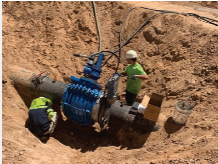
4 Milling the 120° slot across the pipe
