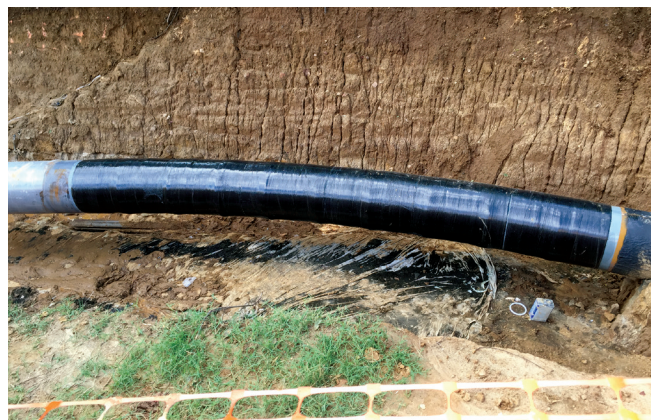
Composites provide quality repairs that can be installed quickly for reliable results. (Photos by ClockSpring|NRI)
