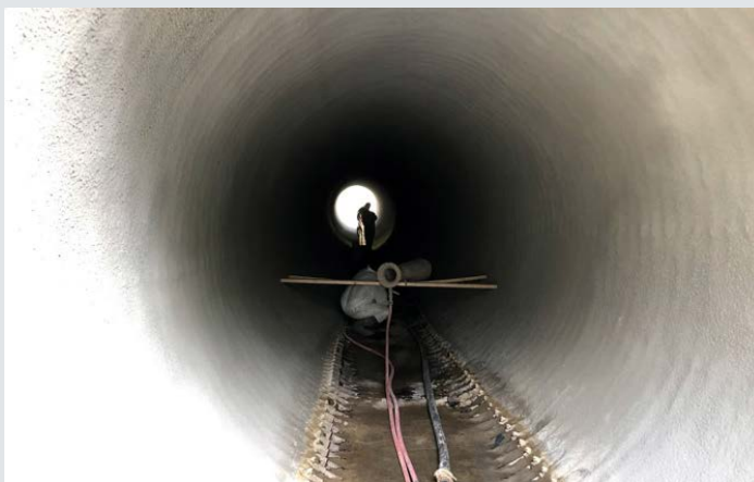
Bottom of pipe left until last for ease of install.
