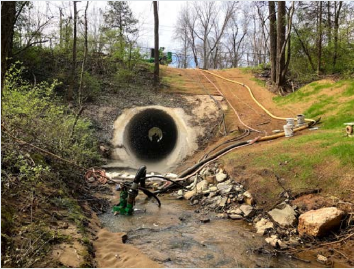
Bypass set up - Paw Creek is a live stream flow
