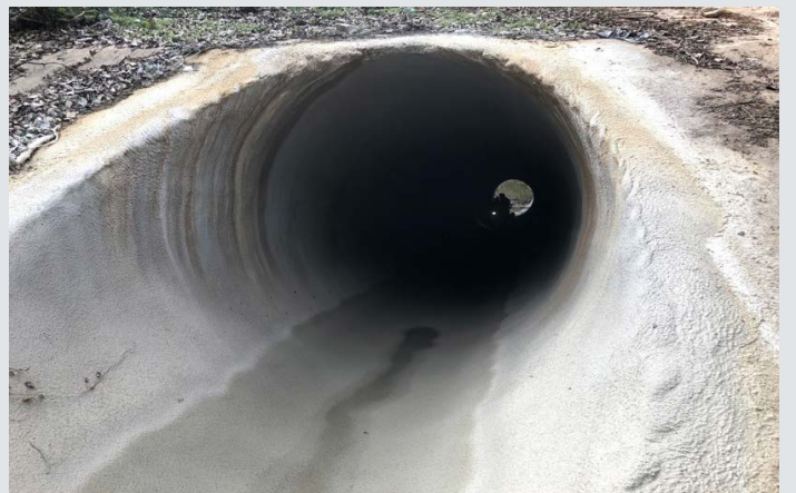
Completed installation of GeoTree GeoSpray.
