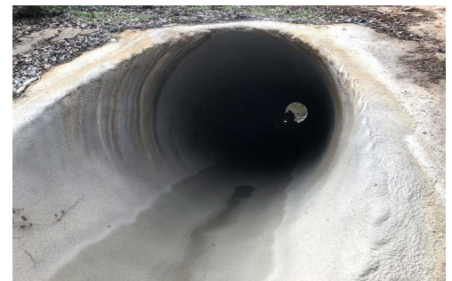
Completed GeoSpray installation.
