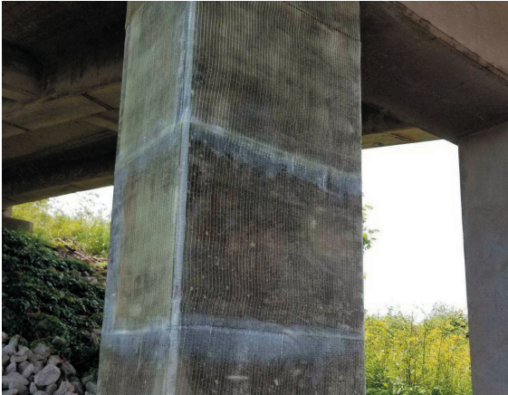
Finished column after wrapping was done
