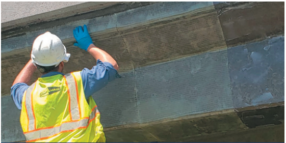
Hydratechs crew installing the Tyfo SEH51A glass fiber
