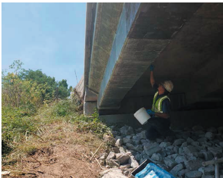
Hydratechs crew installing the Tyfo SEH51A glass fiber
