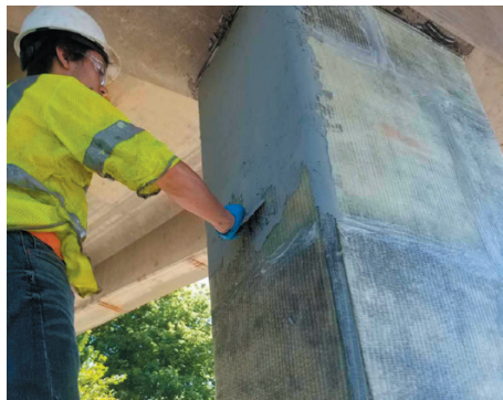
Application of Tyfo RR after the fiber has been applied
