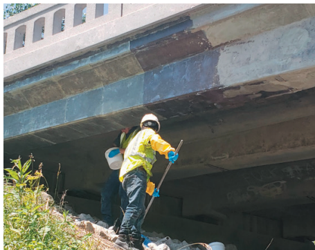
Hydratechs crew installing the Tyfo SEH51A glass fiber
