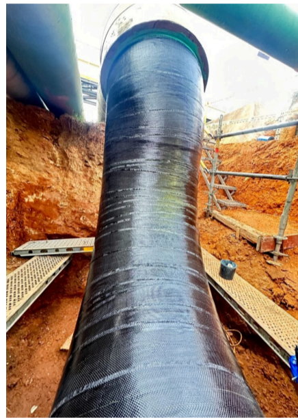
Atlas is applied in a spiral fashion the full length of each repair.
