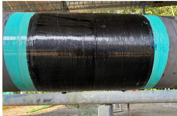
Next, 12 layers of Atlas were applied in an offset manner.
