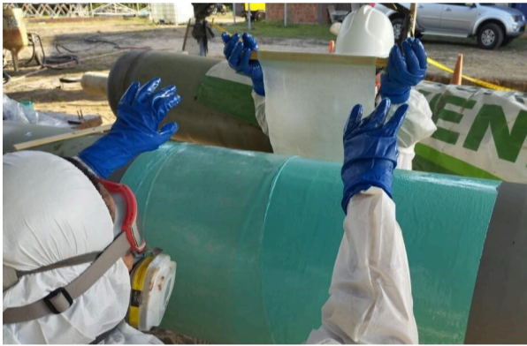
Fiberglass impregnated with SFE 206 was applied over the PPR 290 primer.
