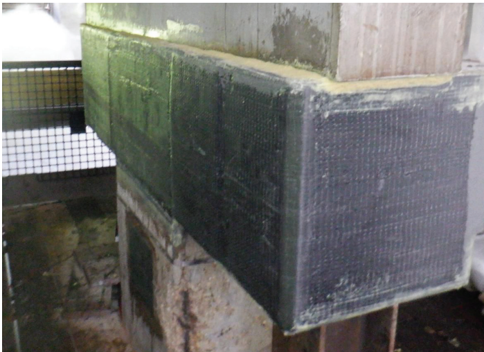
Horizontal layers applied
