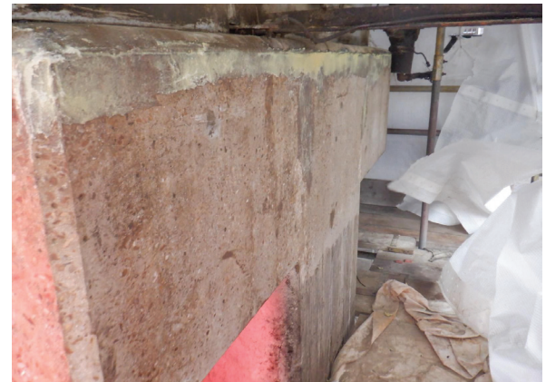
Surface prepared, cracked and damaged areas filled
