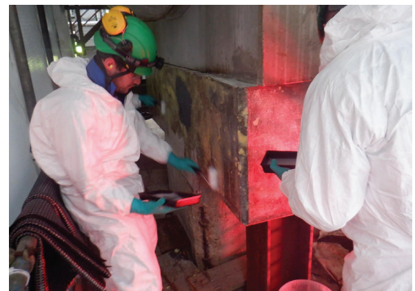
Tyfo S applied to the surface area
