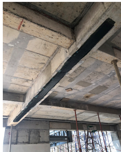
RenewWrap EZ-Slit FRP - cut to size Ready-cut widths of RenewWrap in place
