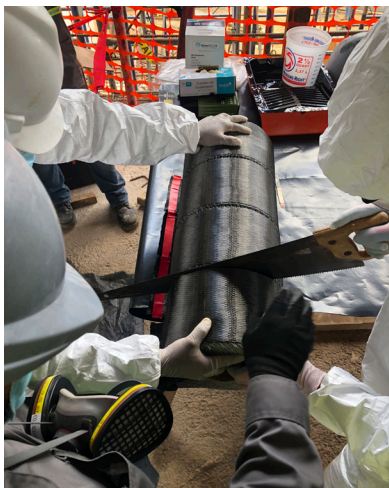
RenewWrap EZ-Slit FRP - cut to size Ready-cut widths of RenewWrap in place
