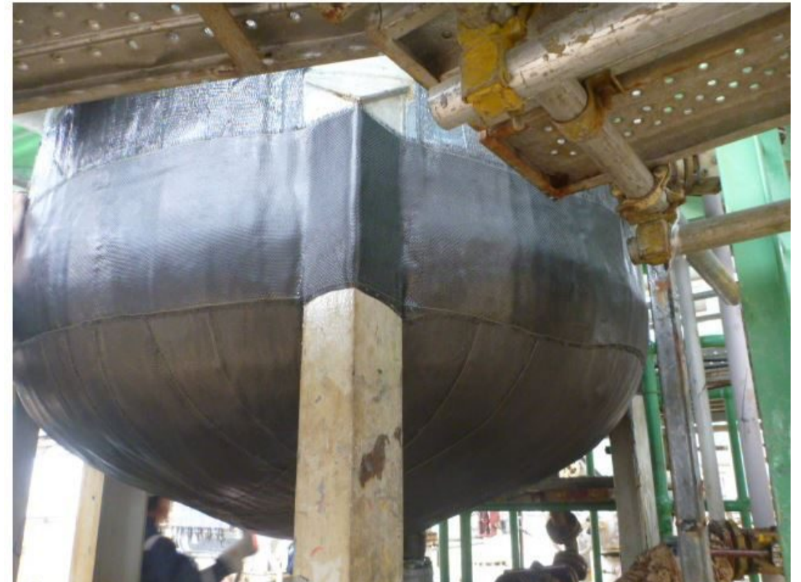
Figure 6: Application of the Atlas™ Repair System
