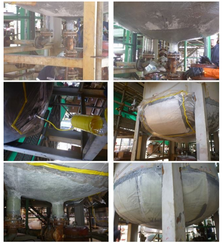
Figure 3: Application of the initial 4 FormaShield™ layers
