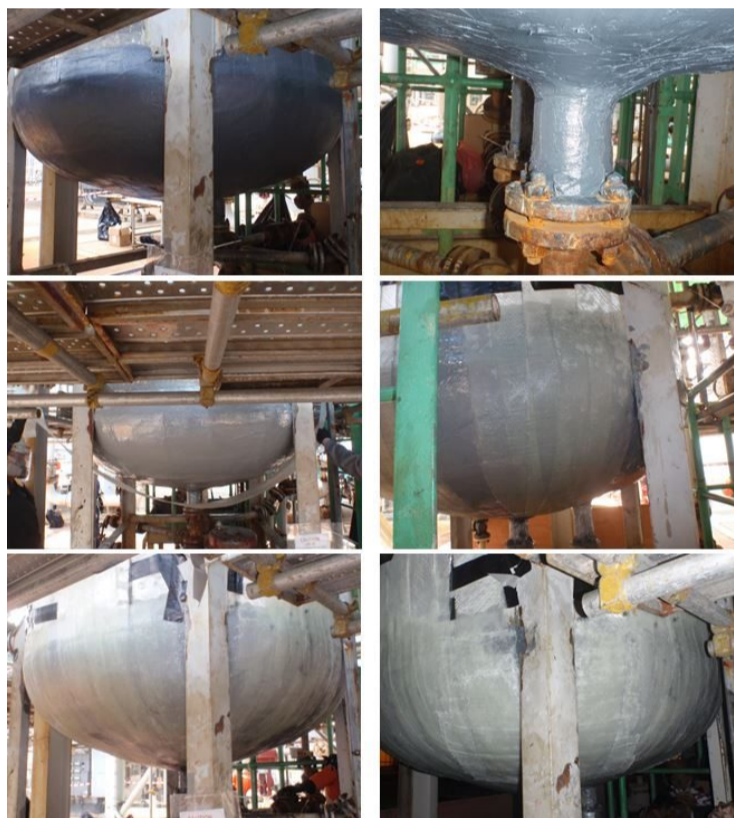
Figure 4: Remaining FormaShield™ Installation
