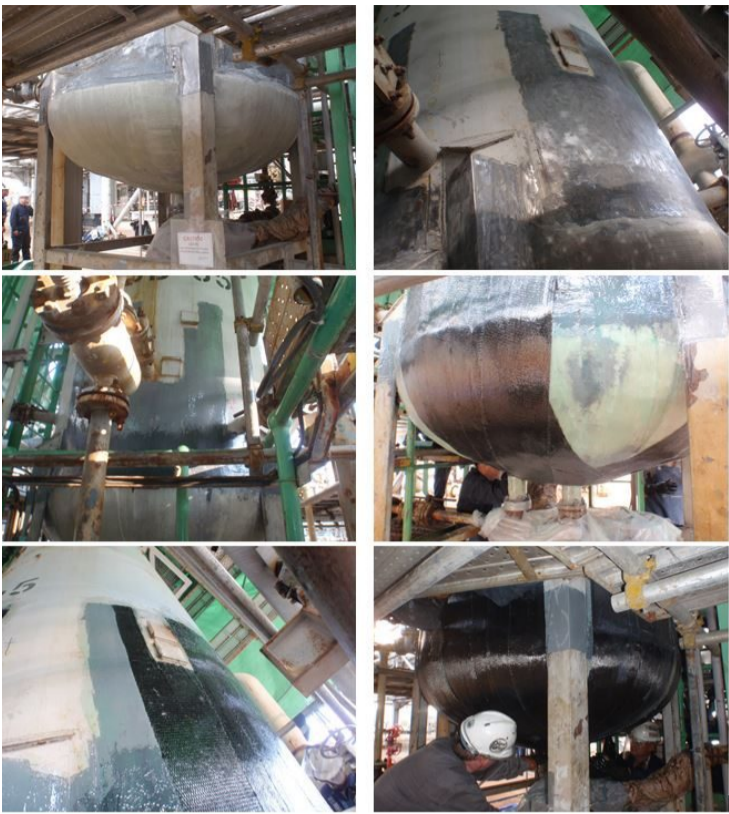
Figure 5: Application of the RenewWrap™ system
