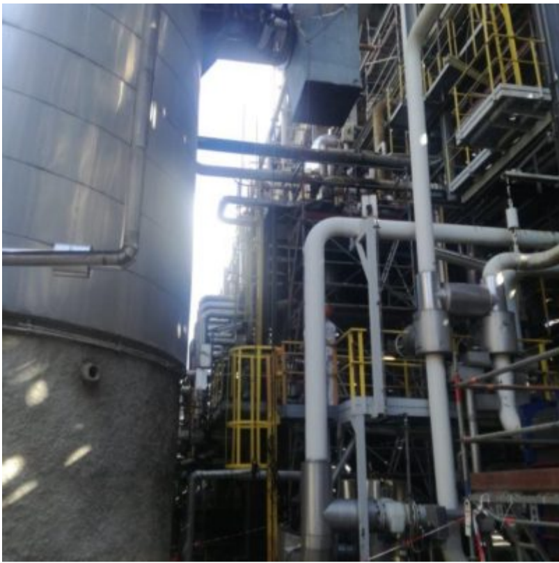
Workers use rope access to inspect the pipe.
