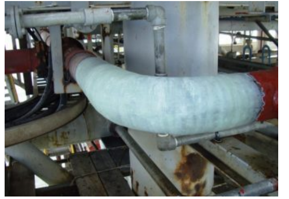
A Contour composite repair restored the damaged line to safety.
