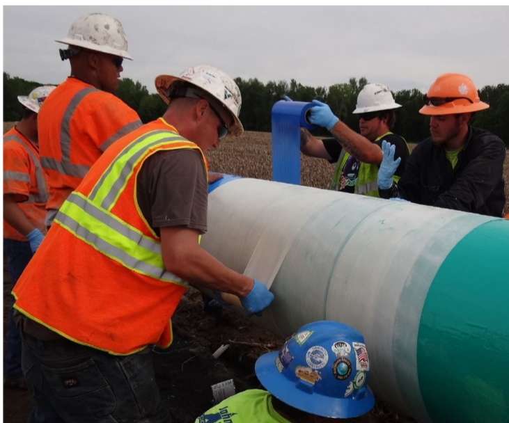
With a successful test pull determined the ARO could withstand the abrasion from the cobble.
