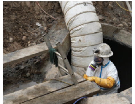
Bypass system installed to divert wastewater around the work area
