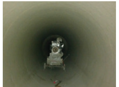
The pipe was sprayed with GeoSpray mortar to a two-inch thickness
