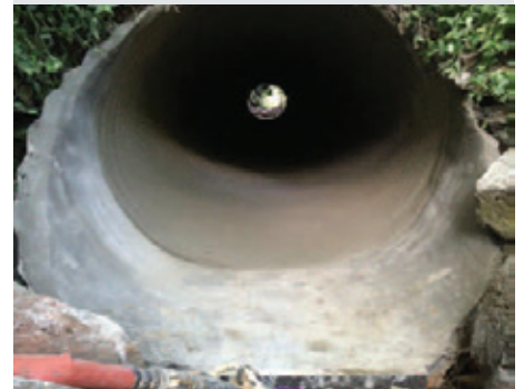
Kashmir Road culvert after GeoSpray mortar rehabilitation.
