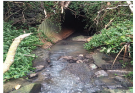
Kashmir Road culvert prior to GeoSpray mortar rehabilitation.
