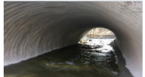
Final structurally-enhanced culvert back in service.
