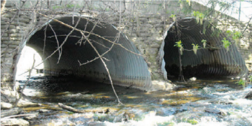
Initial state of culvert outlet prior to rehab.
