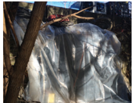
"Tenting" the culvert to protect from the temperature during initial curing.
