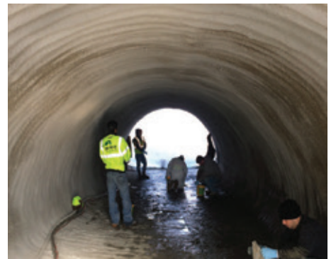
Repair of infiltration in invert after the initial liner application.
