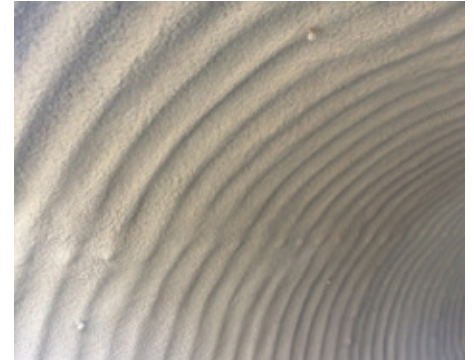
Close-up view of initial passes of geopolymer liner.
