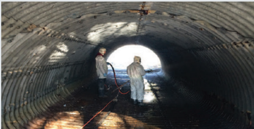
Initial hand-spray application of geopolymer mortar.
